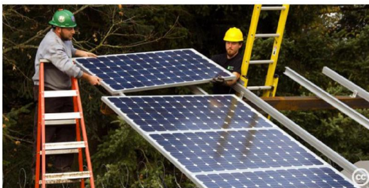
Figure 12: Installing Solar Panels Oregon Dept. of Transportation., Creative Commons License.
