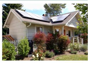
Installing solar panels to face the west in addition to the south can reduce pressure on grid and enable solar power to satisfy a portion of peak afternoon demand. Image credit: NREL/Brothers Electric © 2008
